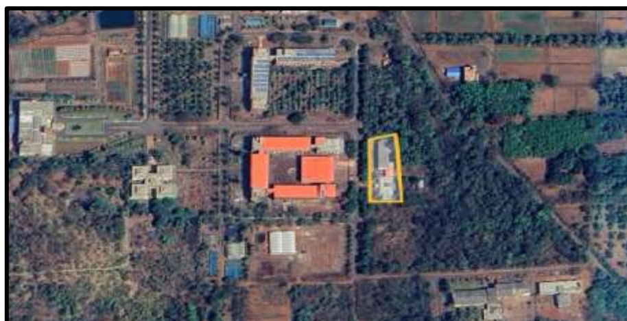
Figure 4. College of Forestry Building-3
